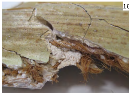
Figure 16: Section through historic fibrous plaster.
