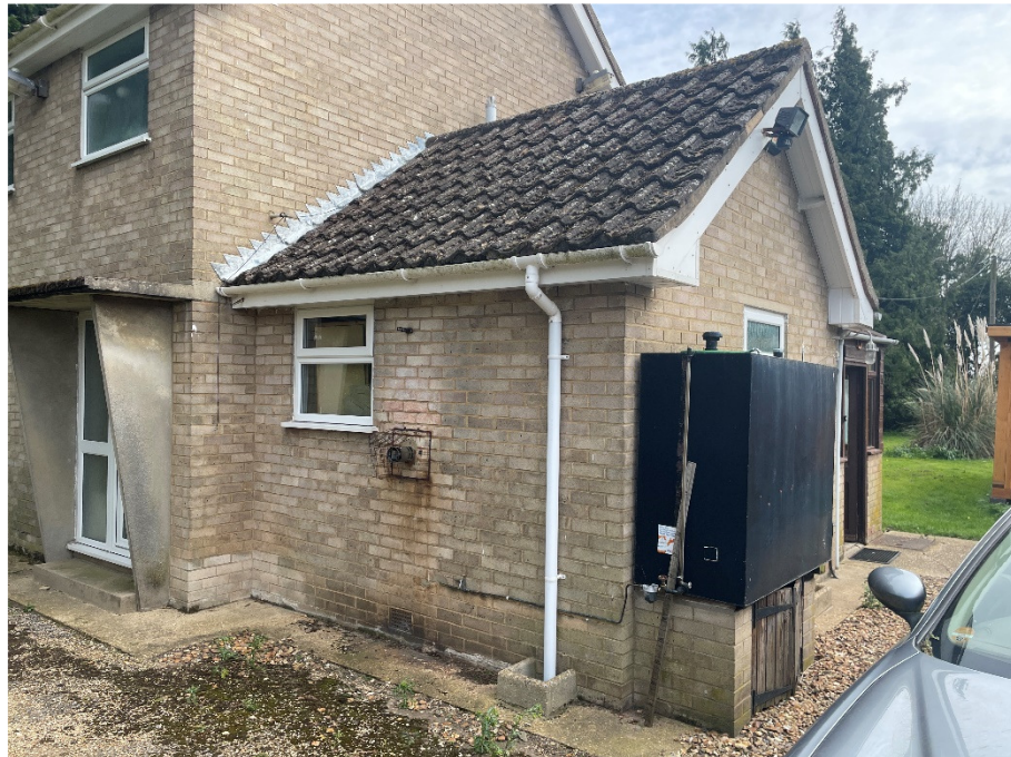
View showing Utility single storey element, with boiler and oil tank
