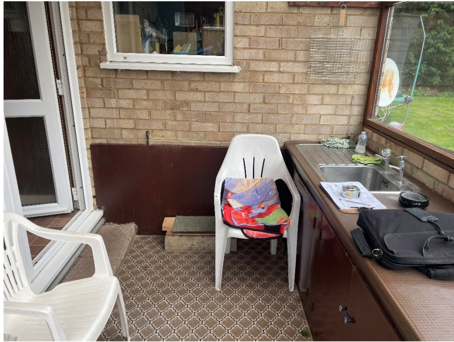
View showing internal view of Conservatory
