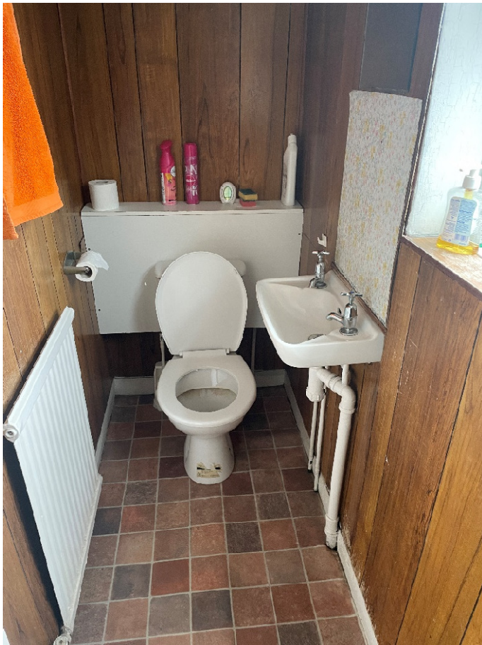
View showing the Shower Room
