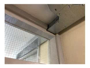
All **trunking** to be fixed directly to the wall where possible. A short piece of lid is to be fixed to the trunking with rivets and the lid is to protrude a maximum of 40mm from the structure on each side. Also a Fire Barrier is to be fitted within and around the trunking once the cables have been installed, such as the Fire Cushion ref: CP651N, Expanding Fire Seal ref: CP660, etc. tested to BS 476: Part 20: 1987 or equivalent. **NOTE all fire stopping MUST have 1 hour rating/protection**
