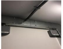
All trunking is to be securely fixed directly to walls or ceilings, run close to ceilings, doorframes and internal corners of walls. There is to be no spacing off the walls or ceilings of the trunking unless specified.
