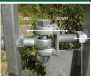
Undoing the nuts on either side of the hang post on this threaded enables you to move the pivot point assembly nearer the hang post (slower) or further away from the hang post (faster) By adjusting the position of the pivot point in relation to the bottom hinge the gate will either close more quickly or more slowly.
