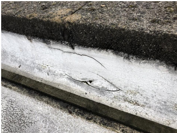
Cracks have formed in the asphalt particularly at the waterproofing upstands.
