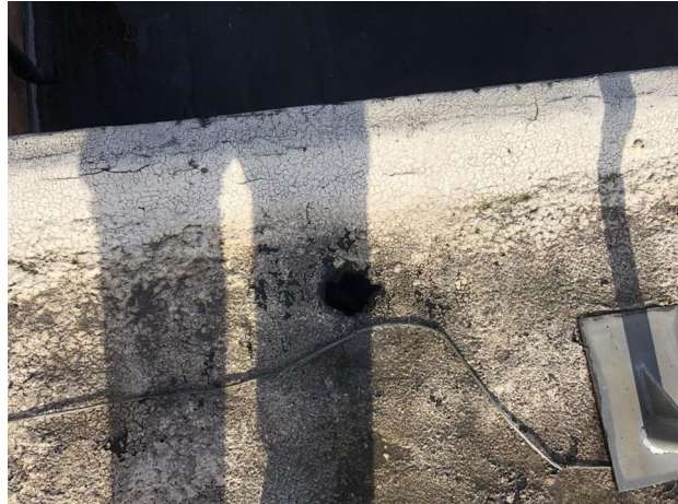
These outlets are very narrow and have no debris guards.
