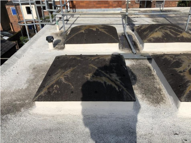
Rooflight kerbs are to be modified and raised to accommodate the insulation levels included within the waterproofing system.
