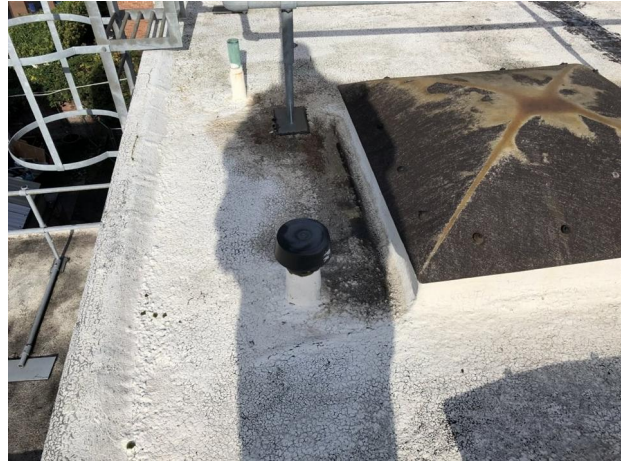
Soil and vent pipes will also need to be modified and raised.
