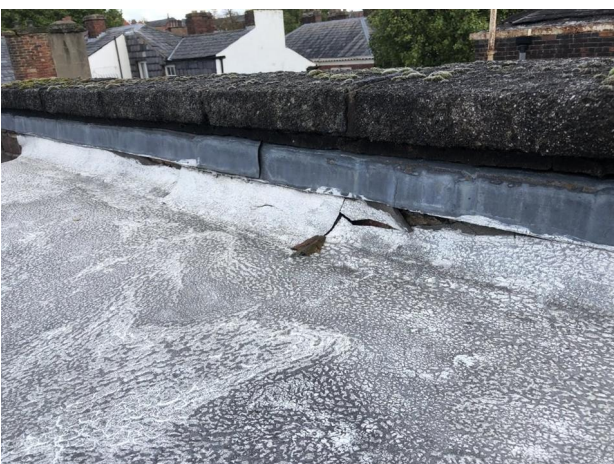
Cracks in the upstand resulting in the waterproofing falling away.
