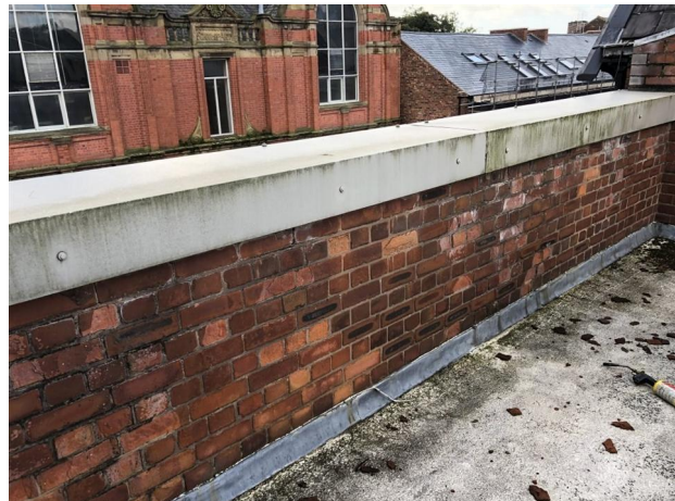
Parapet walls are to be encapsulated in the proposed waterproofing system, subject to conservation approval.
