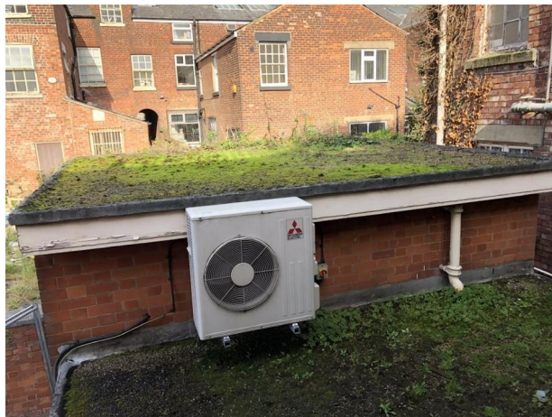
A/C units will need to be temporarily disconnected and raised to accommodate the proposed insulation included within the refurbishment.
