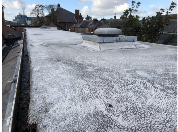
External gutters will need to be replaced and raised as part of the refurbishment.
