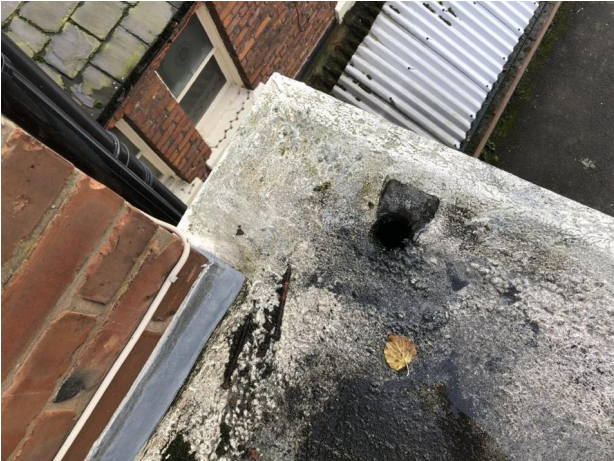
View of typical internal outlet.
