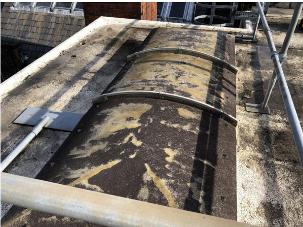
Rooflights are aged and are far below current regulations.
