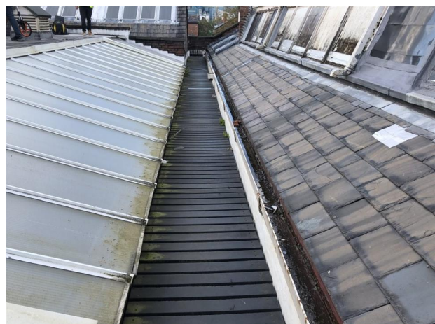
In a number of locations the waterproofing abuts pitched tiled roof areas. Tiles will need to be removed to enable the waterproofing to be appropriately detailed.
