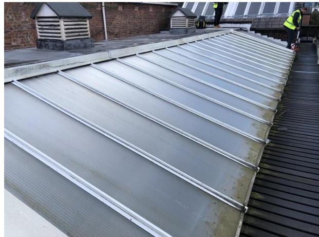
Monitor glazing is also aged and glazed with georgian wired glazing which is below current standard and should be replaced as part of any refurbishment.
