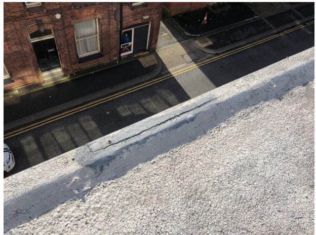
Liquid repairs to perimeter kerb.
