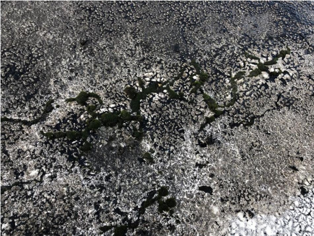
Cracks have formed in the bitumen allowing moss to develop in the cracks.
