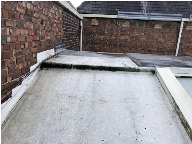
New details to brickwork are to be formed as part of the waterproofing. New secondary flashings are to be introduced.
