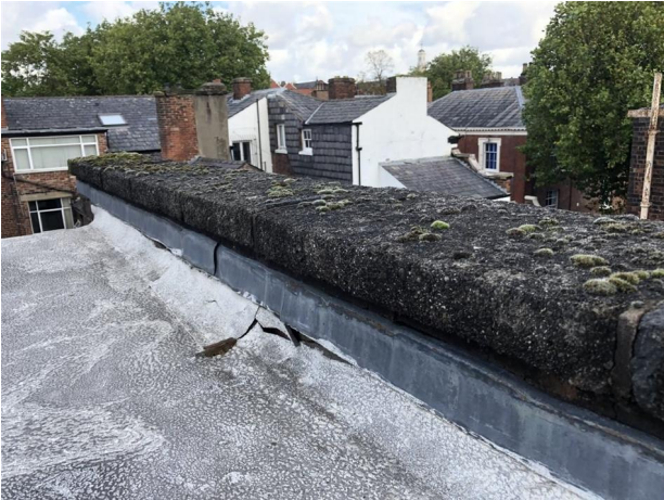
Coping stones are aged and covered in moss. These are to be encapsulated with the new waterproofing system as part of the proposed refurbishment.
