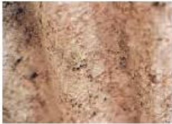
Sprayed coatings on ceiling walls, beams/columns
