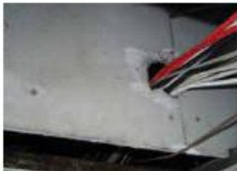
Asbestos insulating board panels
