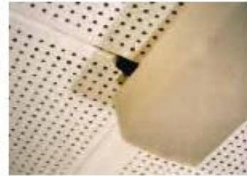
Asbestos insulating board ceiling tiles
