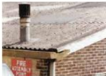
Asbestos cement roof
