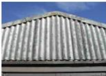
Asbestos cement wall panel
