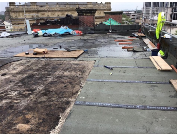
Photo 5 - View of roof 1
