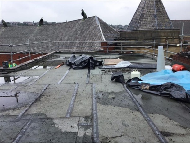
Photo 3 - Overview of progress to roof 1 and falls
