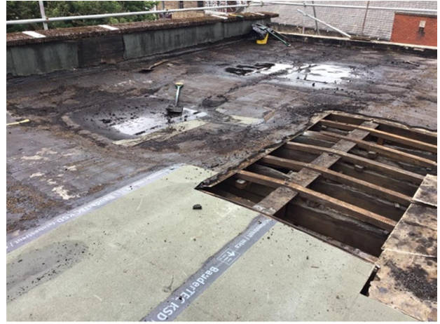
Photo 4 - View of area to be re-joisted
