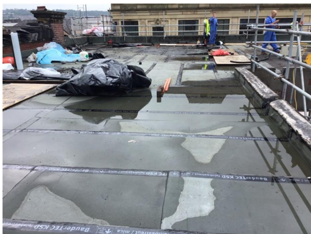
Photo 1 - View of progress to roof 1
