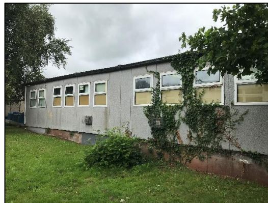
8. Portacabin northwest elevation.
