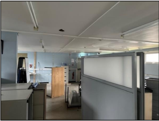
11. Portacabin building internal.
