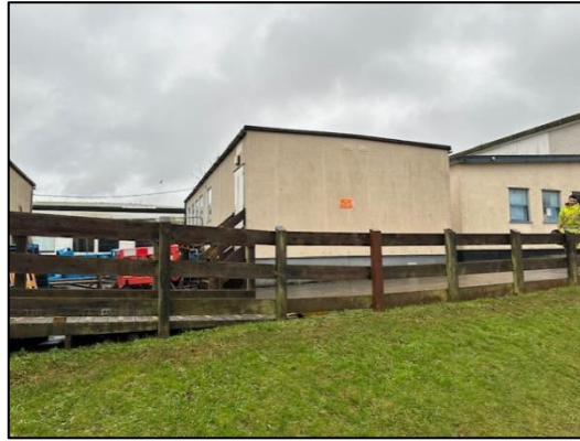
2. Portacabin northeast elevation.
