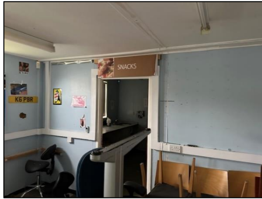
12. Portacabin building internal.
