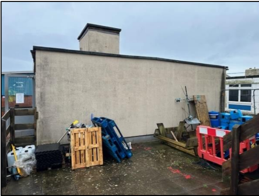
3. Portacabin southeast elevation.
