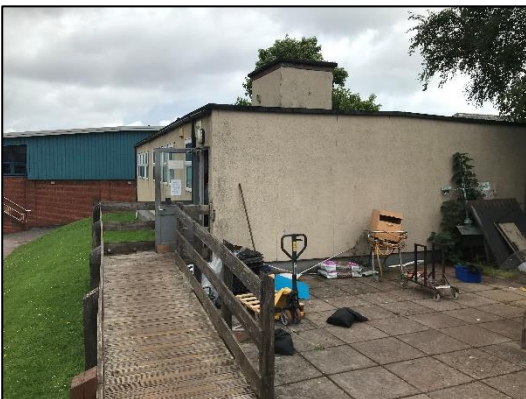
7. Portacabin northeast elevation.
