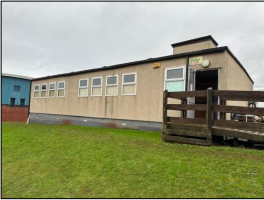
1. Portacabin northeast elevation.
