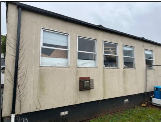
5. Portacabin northwest elevation.
