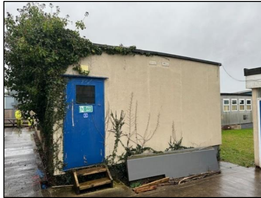
4 Portacabin southeast elevation.
