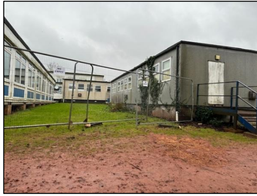
10. Portacabin northwest elevation.
