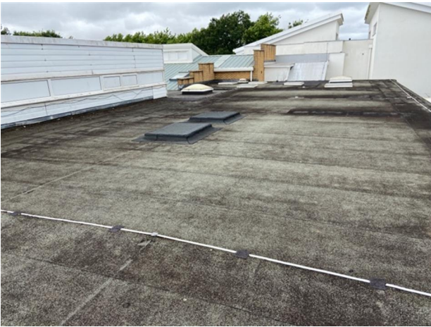
Overview of the roof area
