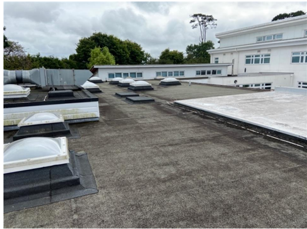
Overview of the roof area
