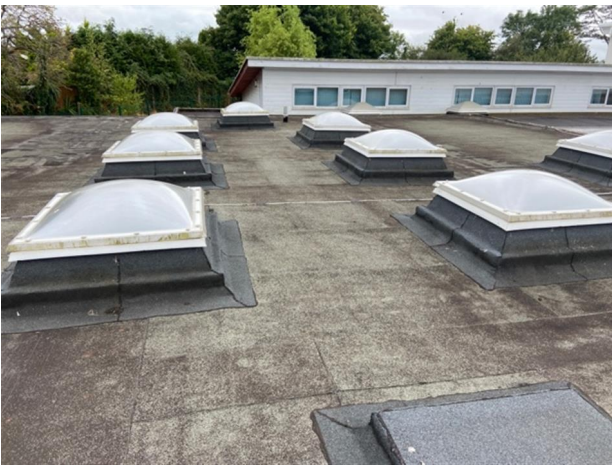
The existing polycarbonate rooflights can remain
