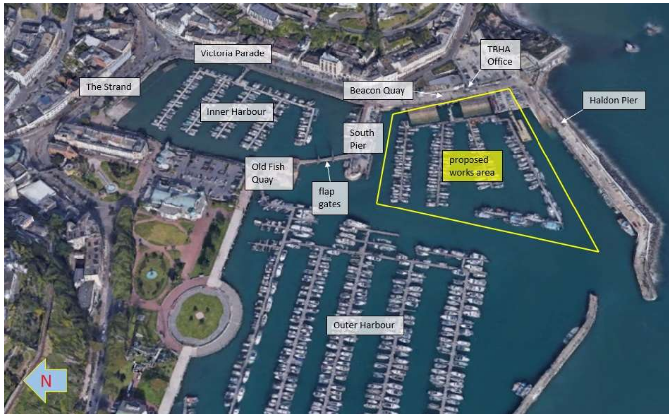
Figure 1 – aerial image of proposed works area, Torquay Harbour
