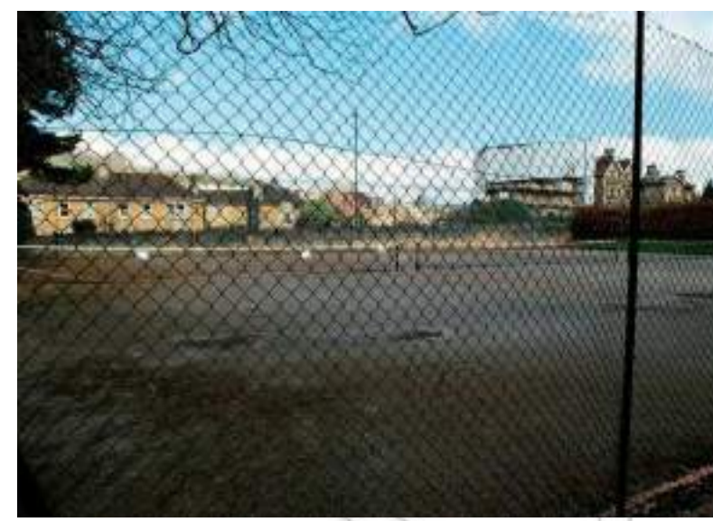
J Tennis Courts Tennis courts in need of repair, multiple provision within Sydney Gardens
