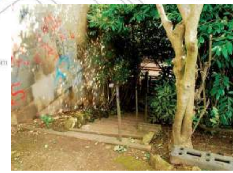
Limited access to railway in parts overgrown
