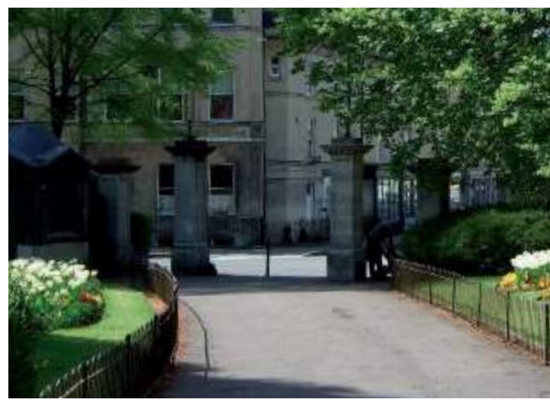
Main Entrance Historic entrance to the park, gates are missing. Stonework in need of cleaning and repair
