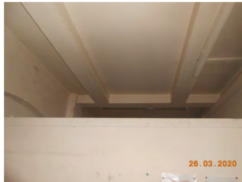
G7 Trimming Beams to Flat Roof Over
