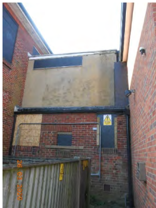
Rear east elevation – 1 st floor infill over single storey
