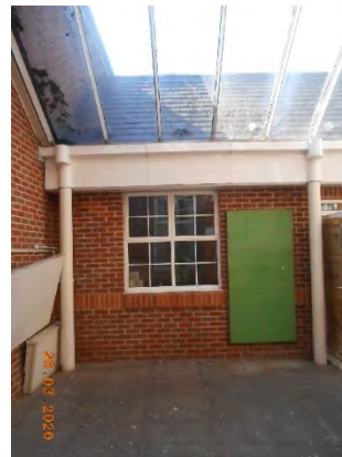
G5 support to glazing at front
