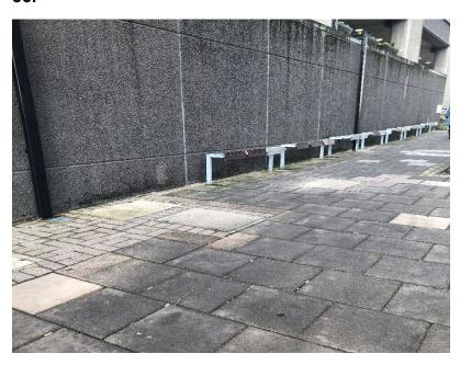
36. This is a frame of the left-hand side of BCC. Again algae and moss and water staining can be seen. More seating here, this being the side most used by smokers. Path on this section is mix of different coloured paving slabs and block paving
