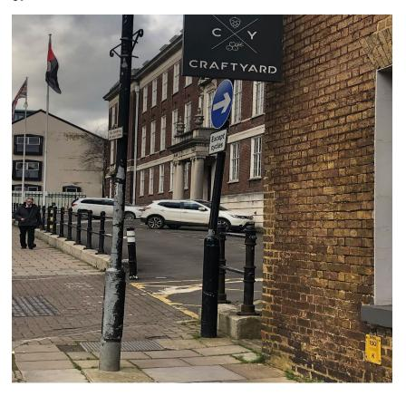
9. First of decorative lamp-posts – this is degraded with paint peeling off. On the floor by the lamp-post is a further Utilities access, with another at the exit point of the car access outside Old County Hall.
