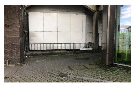
25, 26, & 27, Showing different views of the same section. Note area is suffering from grass/weeds growing through block paving and outlet in concrete wall has algae on the wall. Side access to library or some kind of utility area. Railings need re-painting and boarding is discoloured see frame 26.
