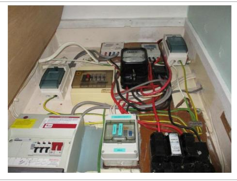
Material Comments: No access gained within electrical boxing due to live status. Presumed asbestos containing flash guards/rope lining within
