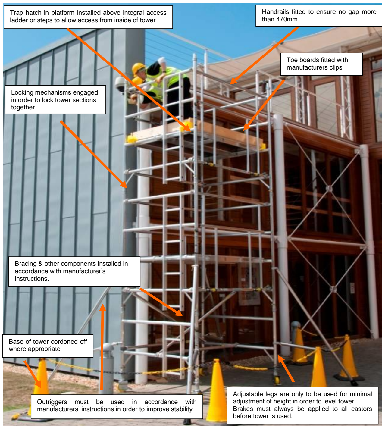
Fig 1 Youngman BoSS Cam-Lock Advance Guardrail system tower, detailing key points to establish when checking
