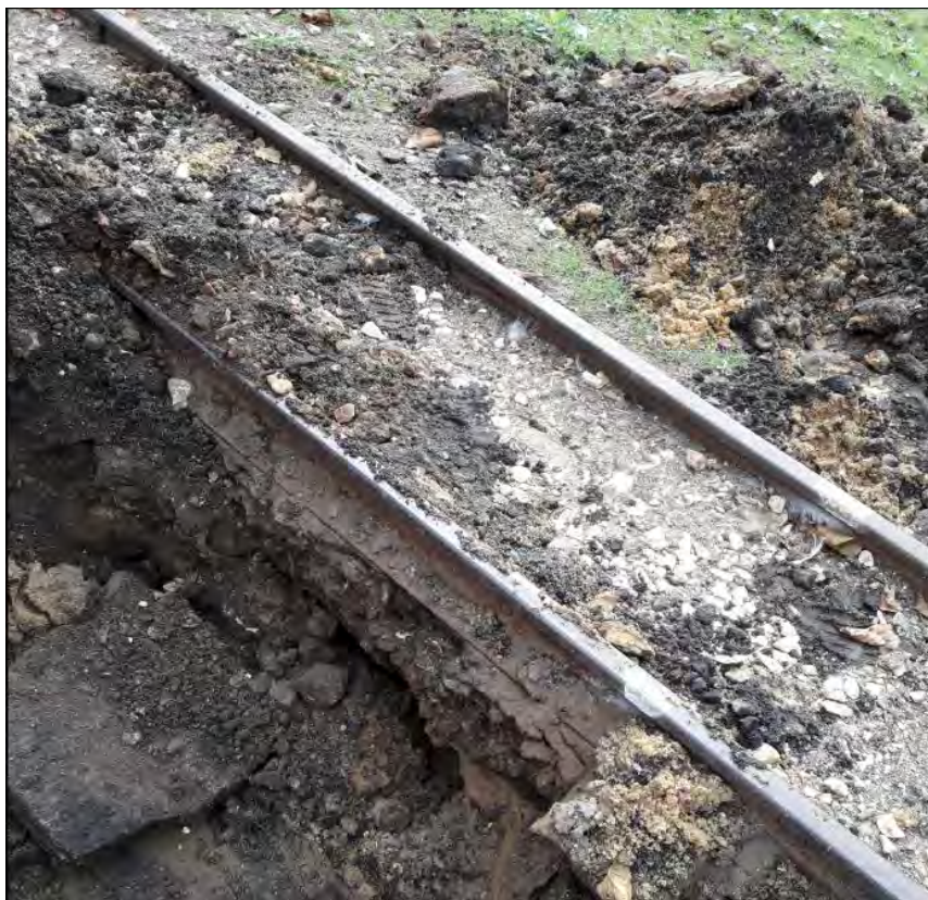
Photo 37: View of the track bed within TP14
