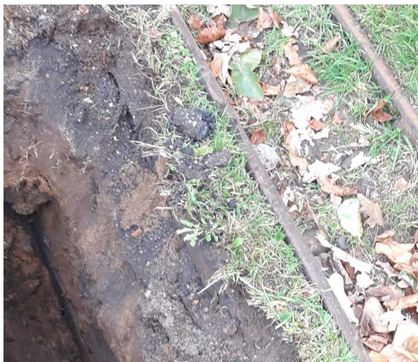
Photo 16: Track bed revealed within TP06
