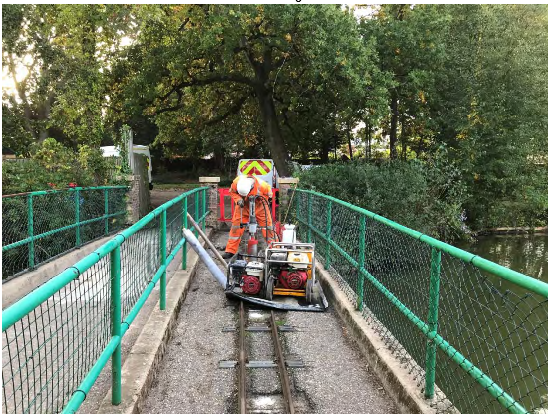
Photo 45 : Coring through bridge deck at location DPA
