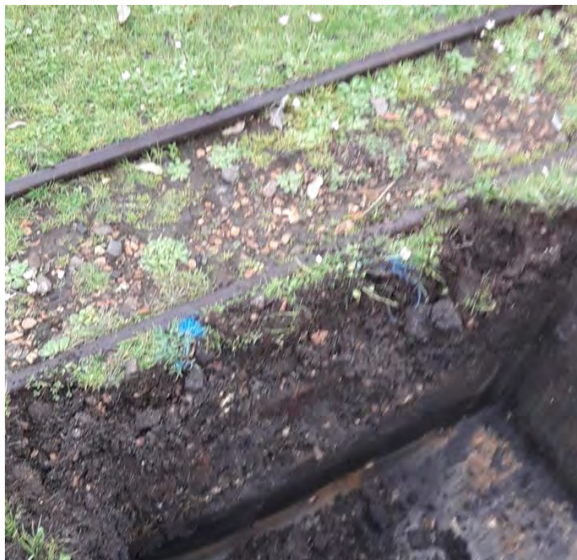
Photo 22: Track bed revealed within TP09
