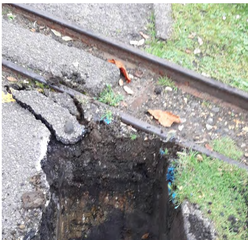
Photo 26: Track bed revealed within TP10
