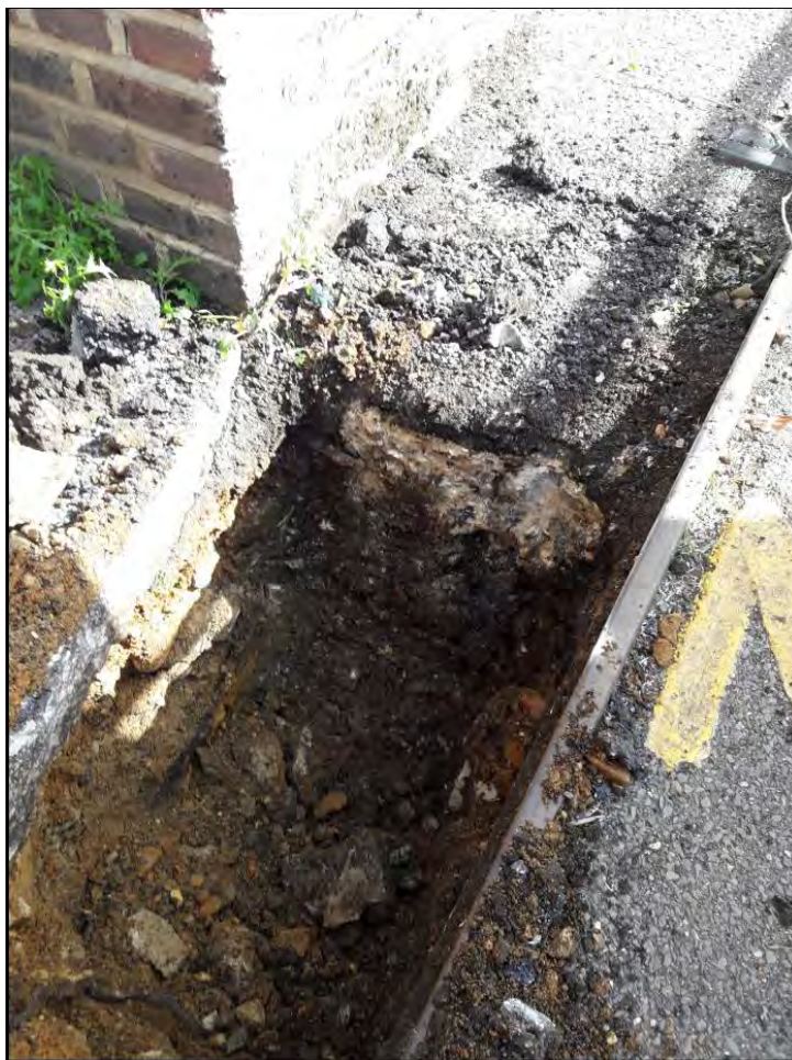
Photo 3: Bridge deck slab revealed within TP01
