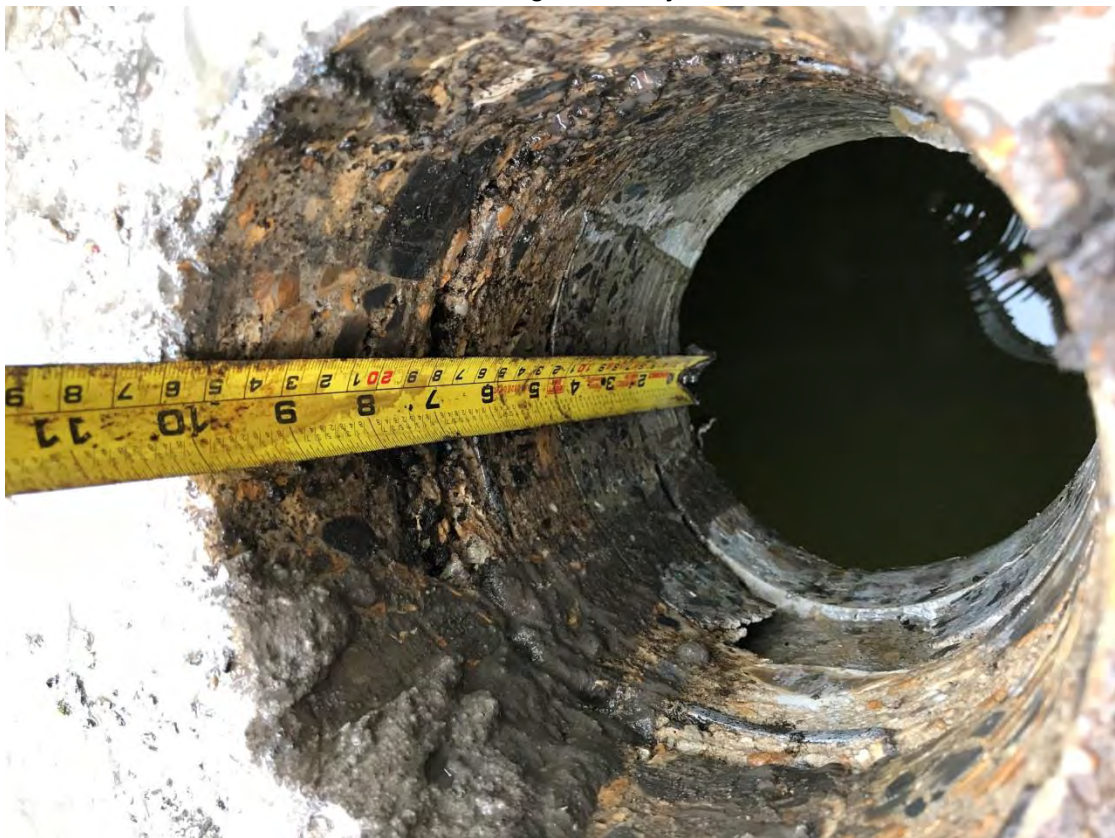
Photo 47 : Core through bridge deck at location DPA
