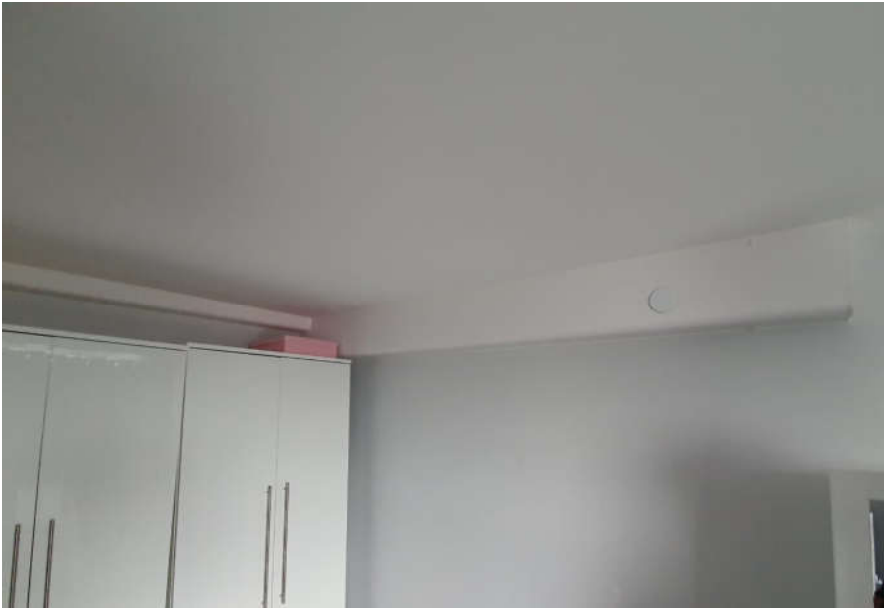
8.2 Typical expectation of proprietary boxing installation within tenanted areas
