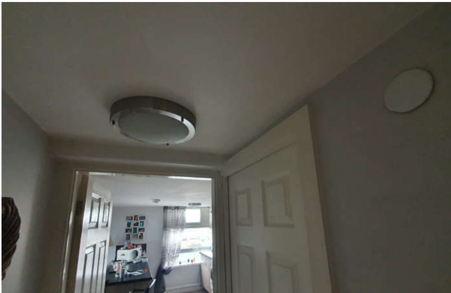
8.1 Typical expectation of sprinkler head penetration in tenanted areas
