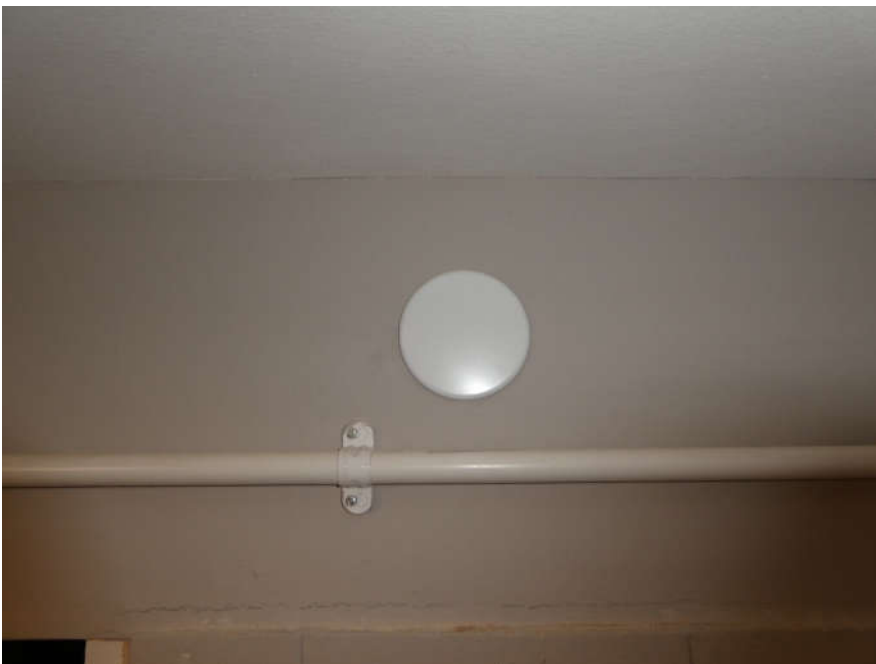
8.5: Typical Upper Floor Circulation Space Sprinkler Head
