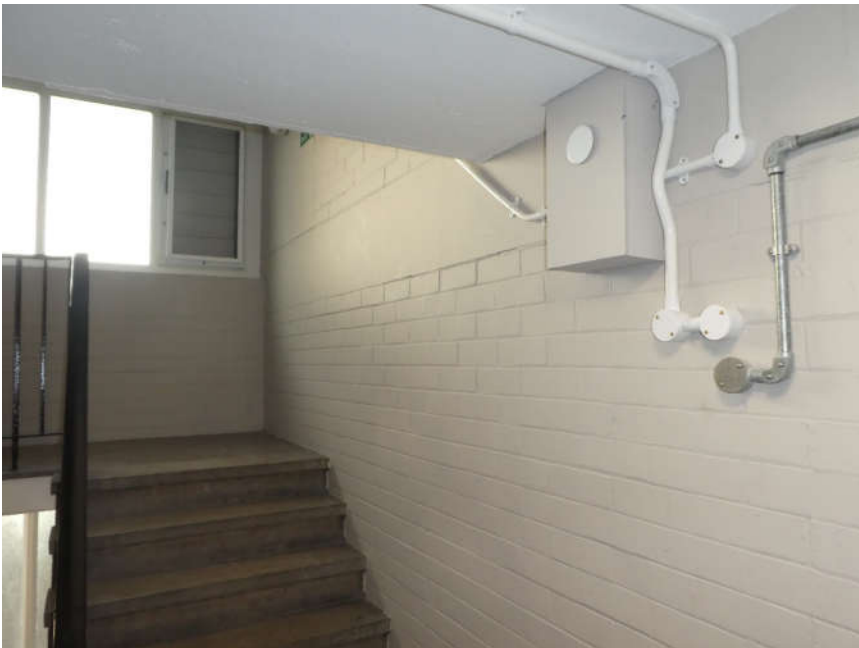
8.7: Typical Stairwell Sprinkler
