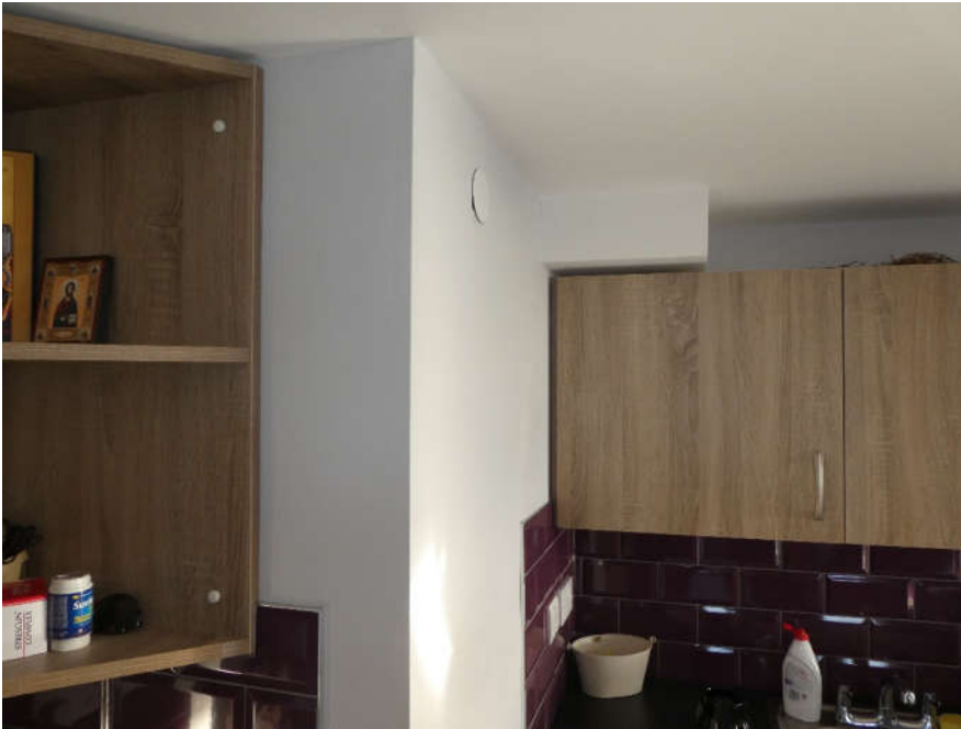
8.4: Typical expectation of sprinkler head penetration in tenanted areas
