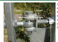
Undoing the nuts on either side of the hang post on this threaded enables you to move the pivot point assembly nearer the hang post (slower) or further away from the hang post (faster)
