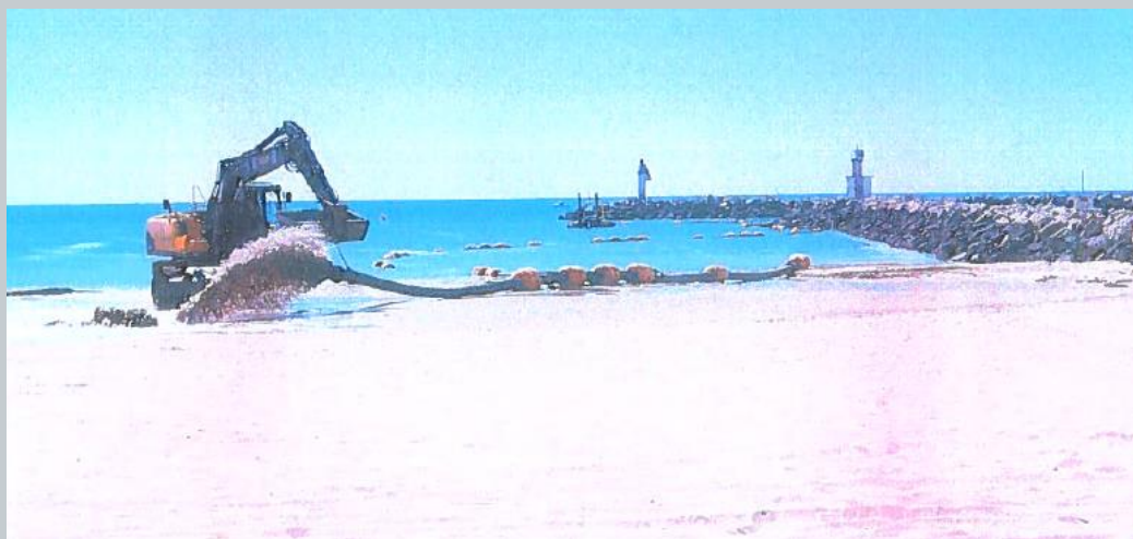
Figure 5 - Example of typical discharge arrangement
