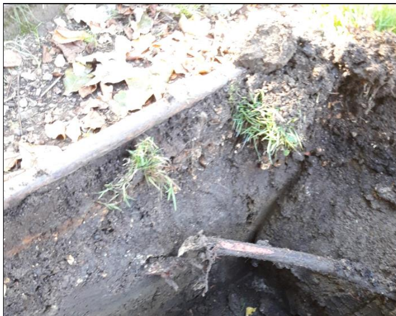
Photo 12: Track bed revealed within TP05
