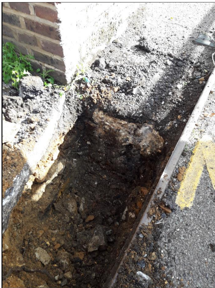
Photo 3: Bridge deck slab revealed within TP01
