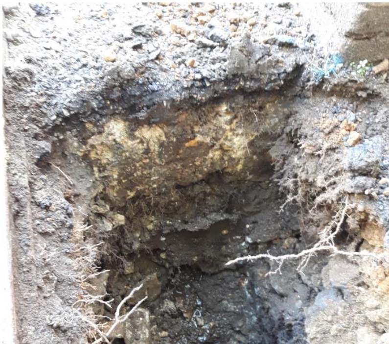
Photo 6: Bridge deck slab revealed within TP02
