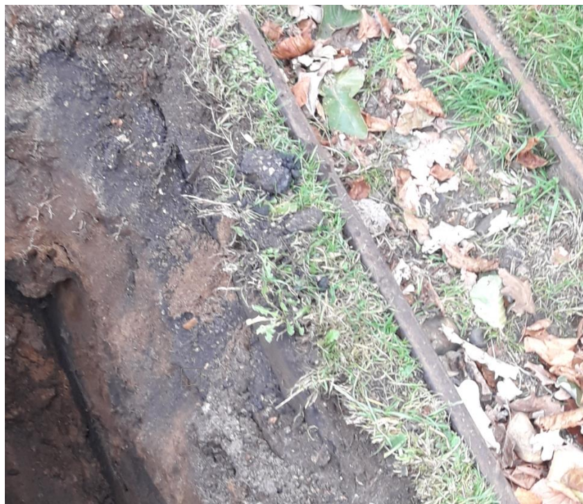
Photo 16: Track bed revealed within TP06
