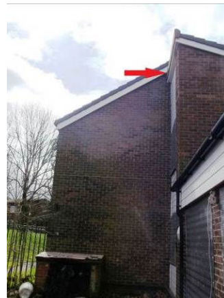
Gable wall of Flat 18 with gap at adjoining structure, and same gable wall as seen from north, indicating location of the gap
