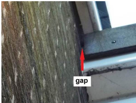
Gable wall of Flat 18 with gap at adjoining structure, and same gable wall as seen from north, indicating location of the gap
