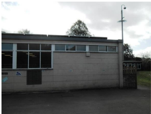
Window Type J – Approx. internal size 2370 x 550mm Total 2 No.
