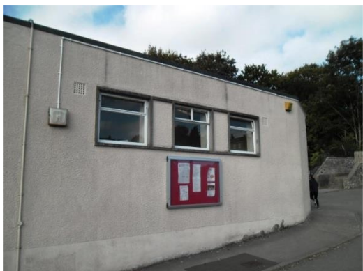
Window Type T – Approx. internal size 900 x 900mm Total 3 No.
