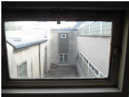
Window Type G – Approx. internal size 590 x 370mm – in glass blocks Total 2 No.
