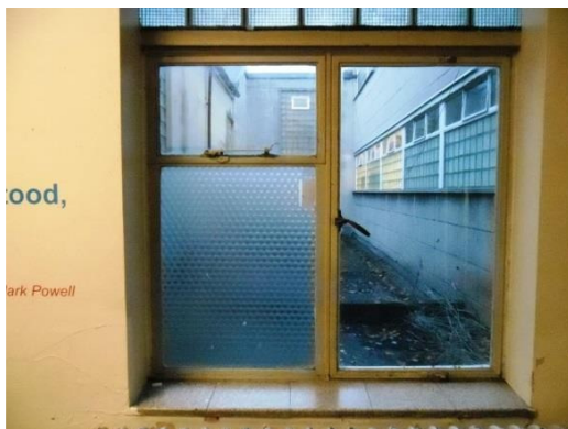
Window Type H – Approx. Internal size 1360 x 1300mm – in glass blocks Total 2 No.
