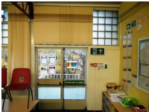
Window Type C - Approx. internal size 2370mm x 1100mm with door approx. 1510mm x 1860mm Total 2 No.
