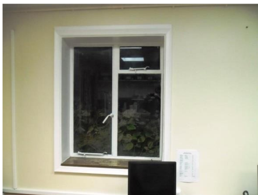
Window Type O – Approx. internal size 1200 x 960mm Total 3 No.
