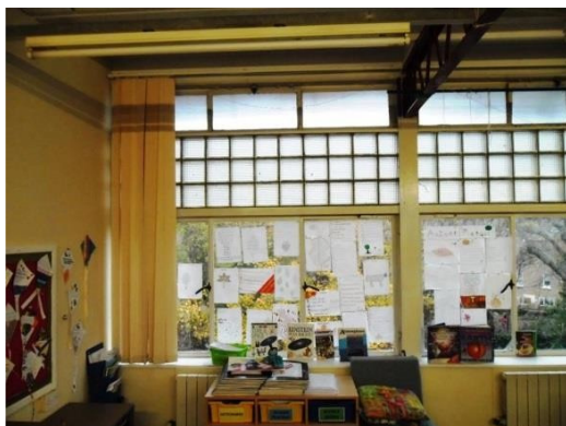
Window Type D - Approx. internal size 2370mm x 2300mm Total 24 No.
