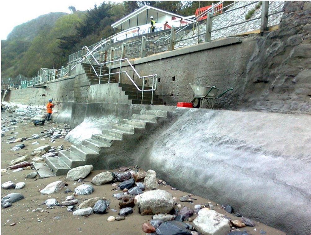
Emergency sprayed concrete works to sea wall, Meadfoot May 2016
