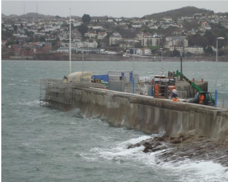
Reinforced sprayed concrete protection to seaward face of Haldon Pier, Torquay
