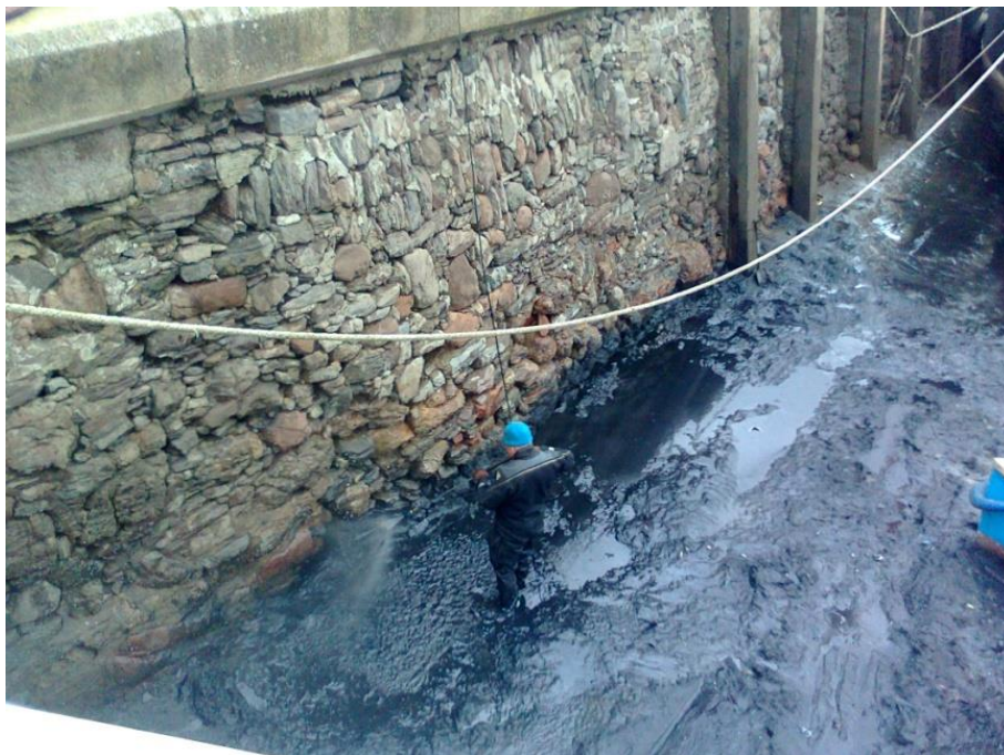
Repair by pressure pointing/grouting of section of bellying masonry, Crane Pier, Brixham
