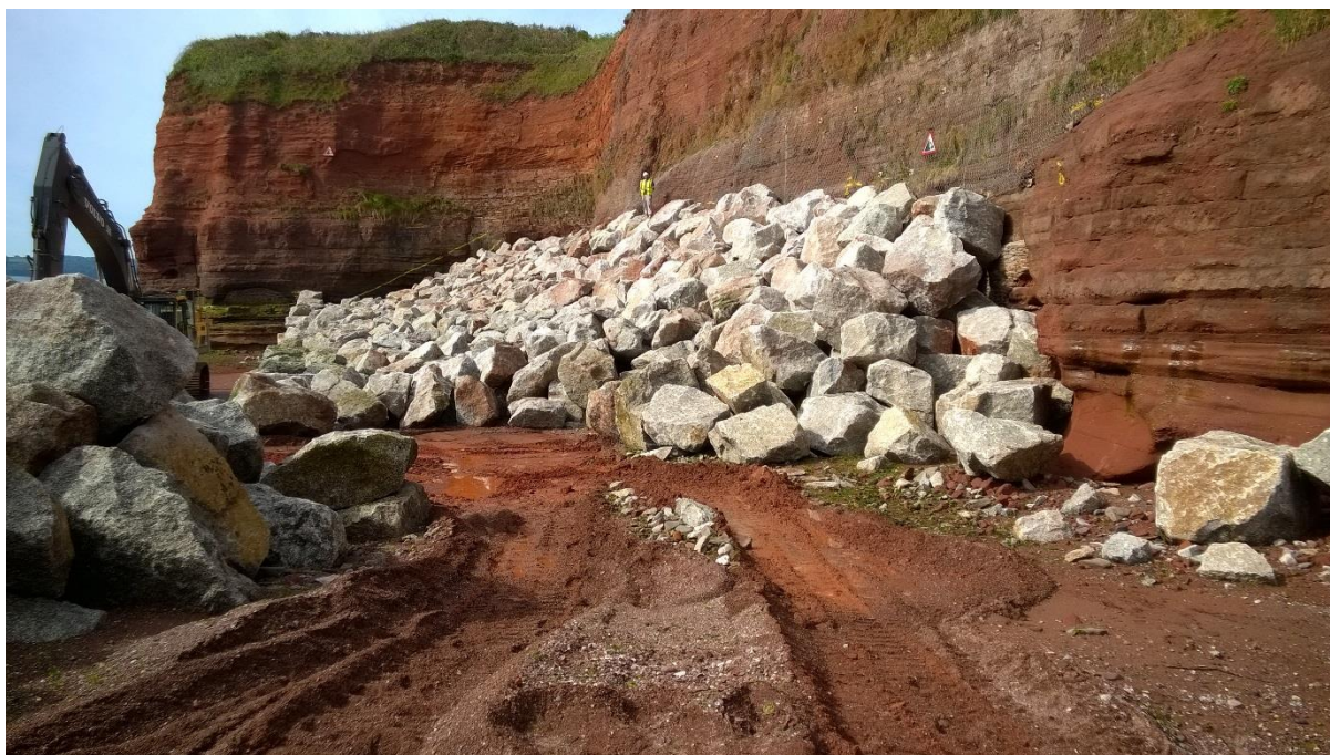
Hollicombe Rock Armour cliff protection May 2017
