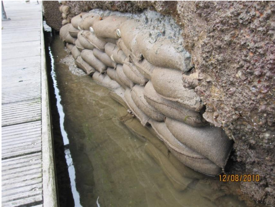
Bagwork and mass concrete repair of scour damage/voids to foundation of Haldon Pier, Torquay
