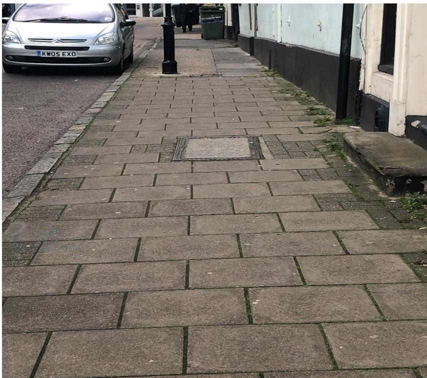
18. Closer image of the pathway detailing utilities access. Again grass and weeds growing through path and gaps from buildings and path
