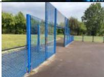
MUGA – Refurbish – repair/replace rusted joints/panels and replace backboards and hoops. Repaint fencing and re-mark.
