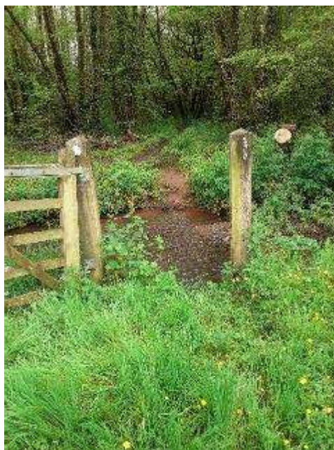
Photograph B: Line of bridge facing east.
