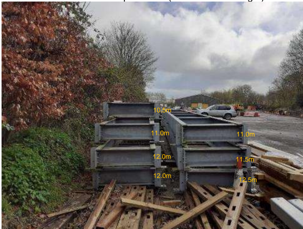
Photo 6 - Stack 2 & 3 with span sizes (+300mm total length) – 06/04/23
