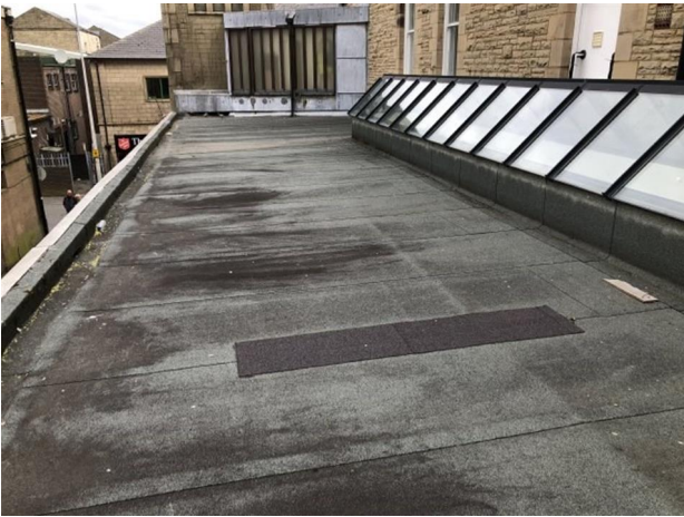
General view of roof area 1 showing the various repairs.
