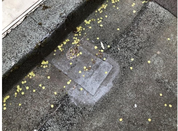
Further evidence of the repairs.
