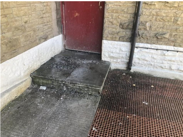
View of the door threshold on roof area 2.
