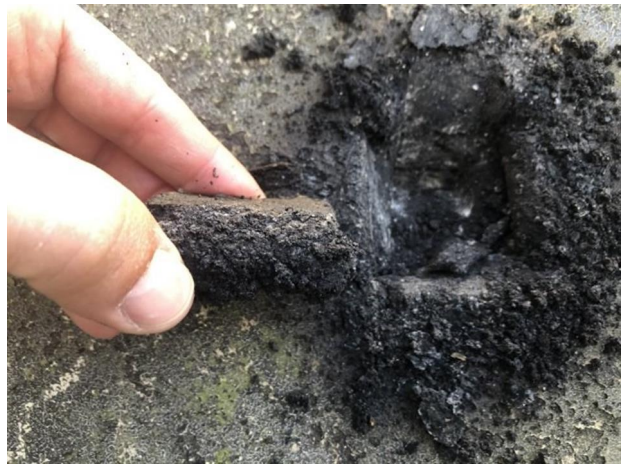
View of the thickness of the asphalt waterproofing.
