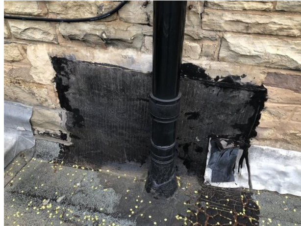
View of the pipe penetration on roof area 1.
