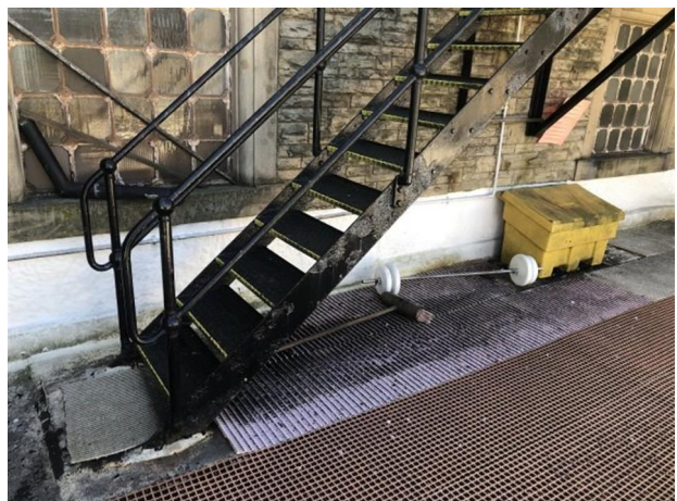
The stairwell will need to be raised temporarily on roof 2.
