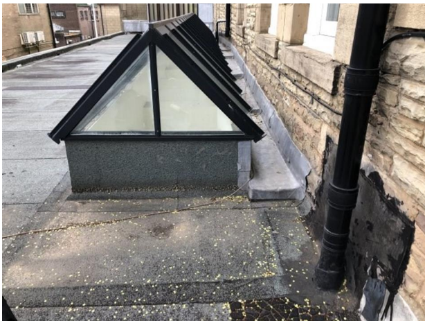
General view of the structural glazing unit on roof 1.
