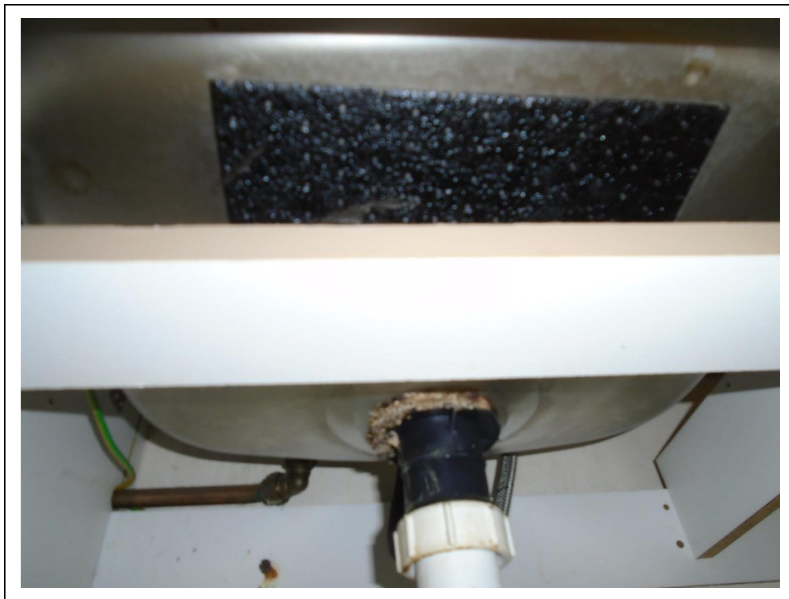
FIGURE 1: CONFIRMED ASBESTOS IN BITUMEN PAD IN ROOM 1, 1/002 - DESCRIPTION & RESULT OF ASSESSMENT (SAMPLE REF. 190316/041019/33)
