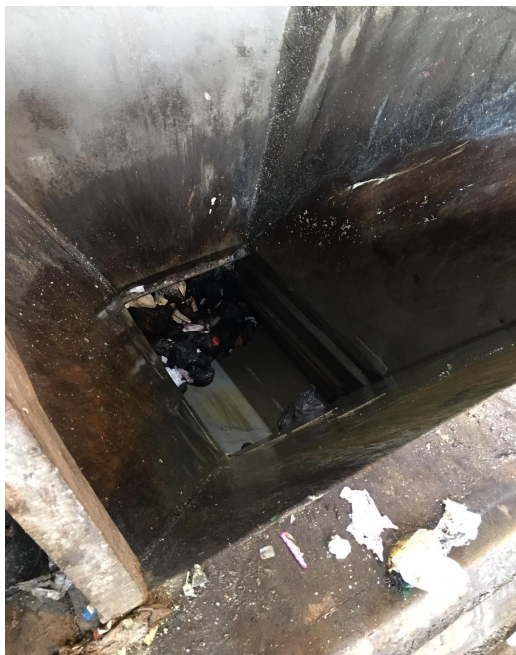
Photo 4 – Patch welding within the hopper
