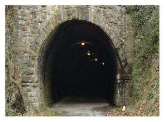
It will be important to keep vegetation cut back close to bridges, tunnels and retaining structures to allow surveyors a clear view of the structure and to avoid damage by any such vegetation, scrub and trees which can cause foundation undermining, masonry to crack and painted surfaces to corrode.
