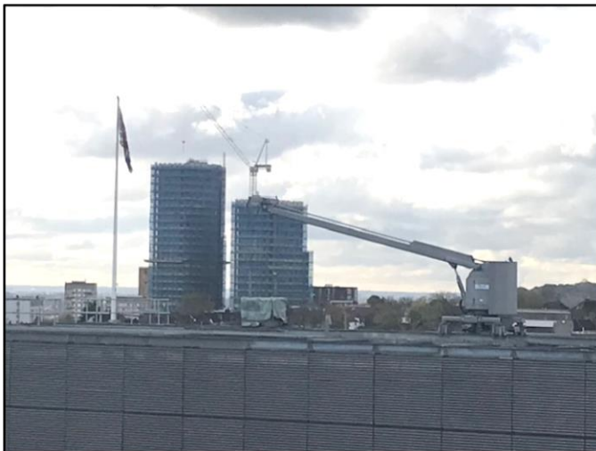
Photo 3a and 3b: Window cleaner basket, which could be used to lift up to roof top level the PV panels (and rails, if using)
