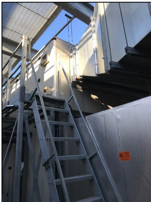
Photo 5: Stairs leading part way up from roof lower (plant) level to roof top level, which can be used to carry PV panels (and rails, if using) part way up to roof top level
