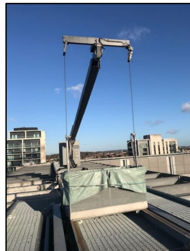
Photo 3a and 3b: Window cleaner basket, which could be used to lift up to roof top level the PV panels (and rails, if using)
