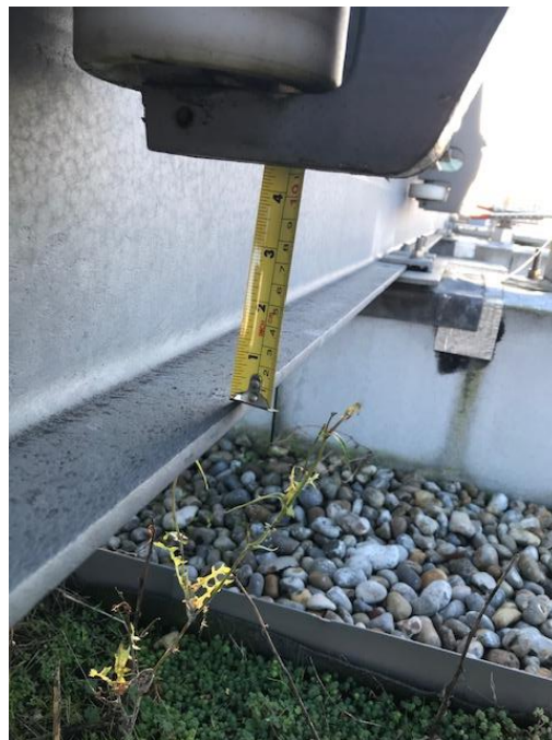
Photo 6: Inner beam, showing overhang of the window cleaner basket, and 10 cm clearance underneath
