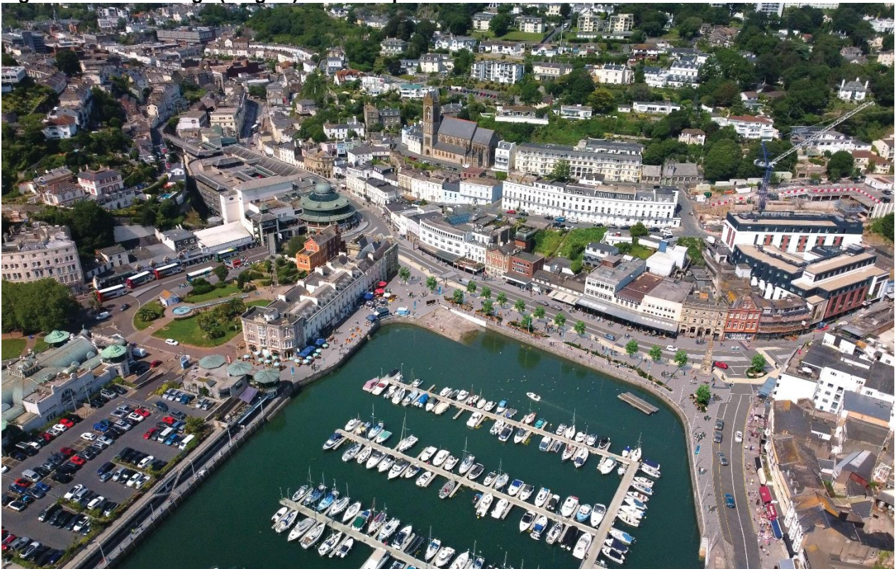
Figure 1.3. Aerial Image (Stage 4) of the Proposed Scheme
