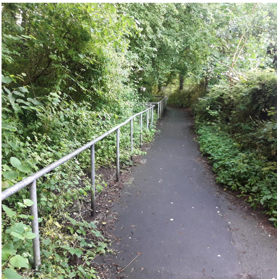
Pic 2 - general view of footpath viewed NE to SW
